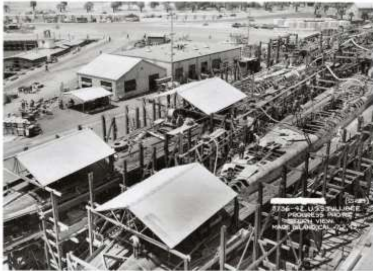
Caption: Tullibee and a sister under construction at Mare Island, 1 July 1942. (U.S. Navy Bureau of Ships Photograph, 19-LCM Box 540, National Archives and Records Administration, Still Pictures Division, College Park, Md.)
